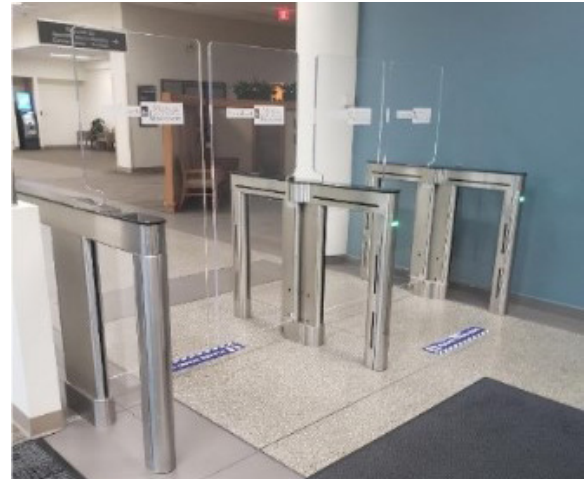
ADA compliant turnstiles at main and staff entrances
